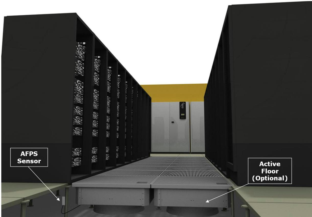
The solution is particularly applicable for Chilled Water installations where the air flow can be adjusted to a very low minimum level (20% on cooling only units). AFPS can also be used on installations for DX systems (air or water cooled) which include multiple Uniflair units.
